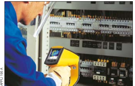
Switchboard inspection
